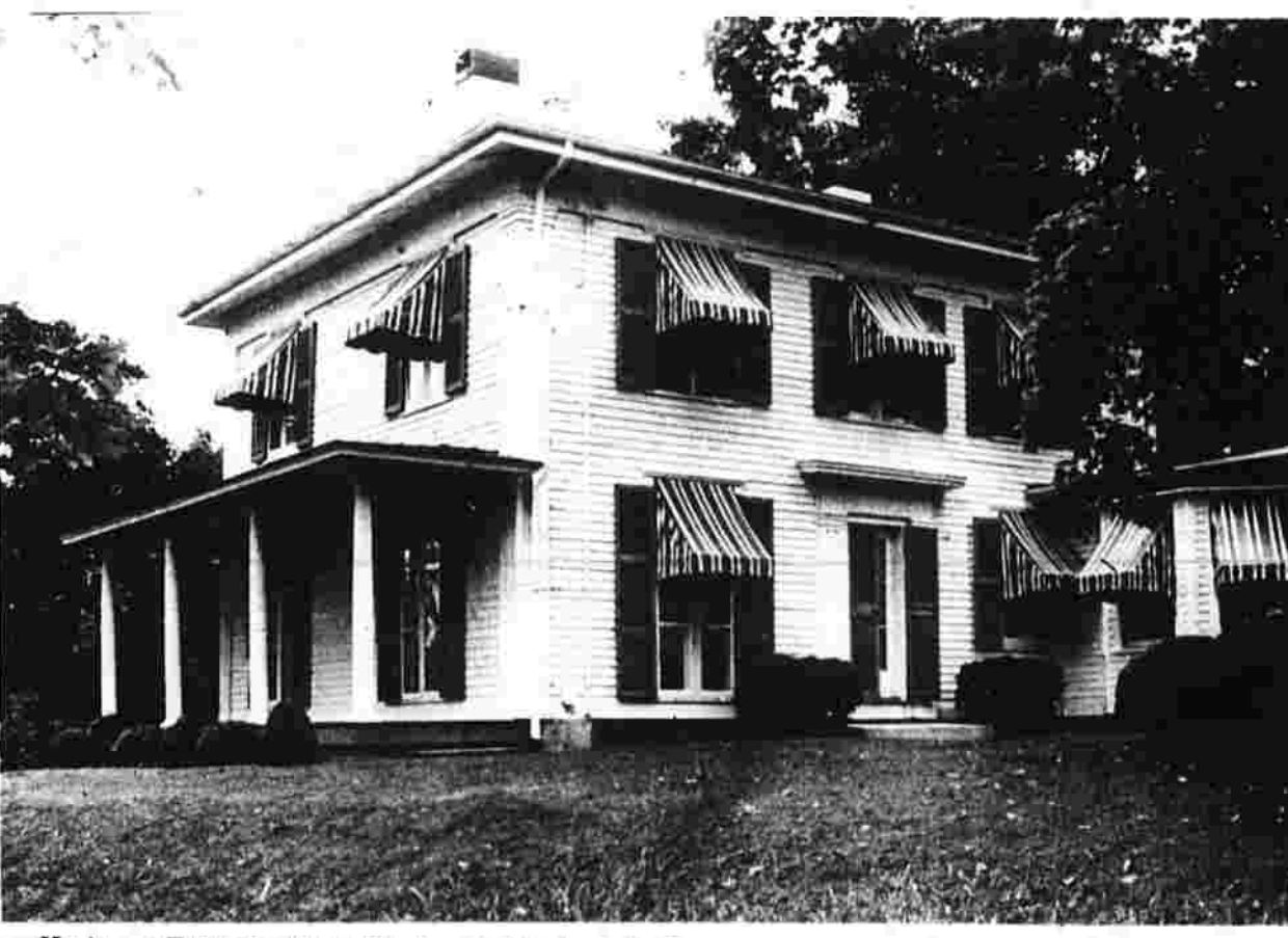
House on E. Center St. built about 1840 by Col. Norman Spencer. A square Greek revival house with center doorway, corner pilasters and an almost flat hip roof. The veranda at the left is probably a later addition.
