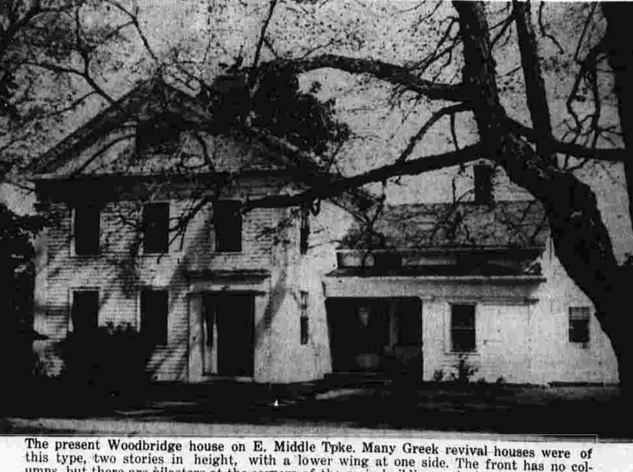
The present Woodbridge house on E. Middle Tpk. Many Greek revival houses were of this type, two stories in height, with a lower wing at one side. The front has no columns, but there are pilasters at the corners of the main building and of the wing, also at the sides of the front doorway. The long narrow windows at the sides of both doorways are typical of the period. Here the beauty of the building lies in its simplicity and its excellent proportions.
