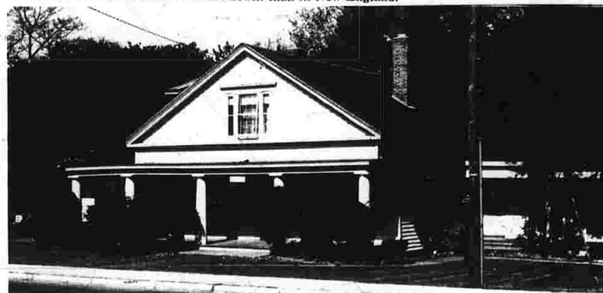
This building, once a Woodbridge house, now serves as a office for the Community Baptist Church on East Center St. It was originally a story-and-a-half Greek revival dwelling, with Doric columns at the front and a wing at one side. The front colonnade has now been extended to the left to enlarge the veranda and a dormer has been added upstairs (left edge of the roof).
